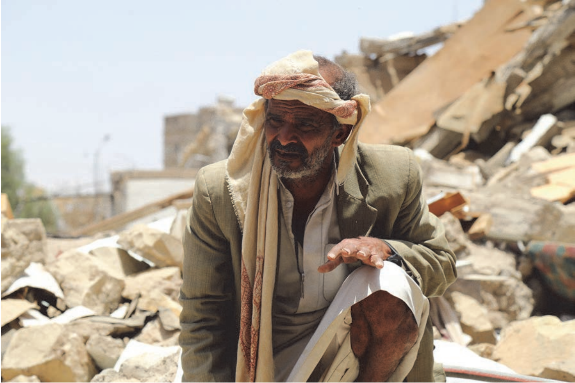
Ayed Ayed Kamil, a neighbor, sits on the ruins of al-Ibbi house, which was struck in an aerial attack on May 5, 2015. © 2015 Ole Solvang/Human Rights Watch
