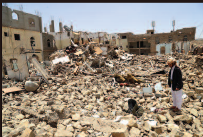
Rubble from a residential house in Saada City. An airstrike almost completely destroyed the house on May 5, 2015, killing 27 members of one family.
