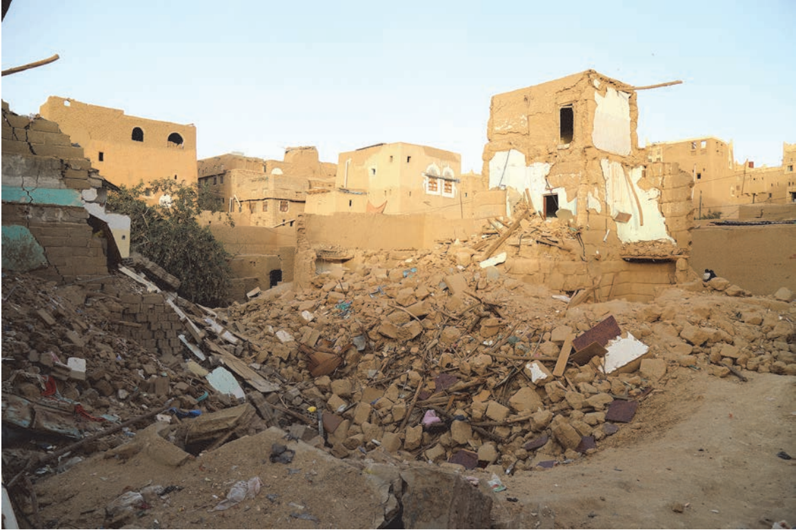
Remnants of al-Sabra's house, which was struck by an aerial attack on April 15, 2015, which killed a woman and her three children. © 2015 Ole Solvang/Human Rights Watch
